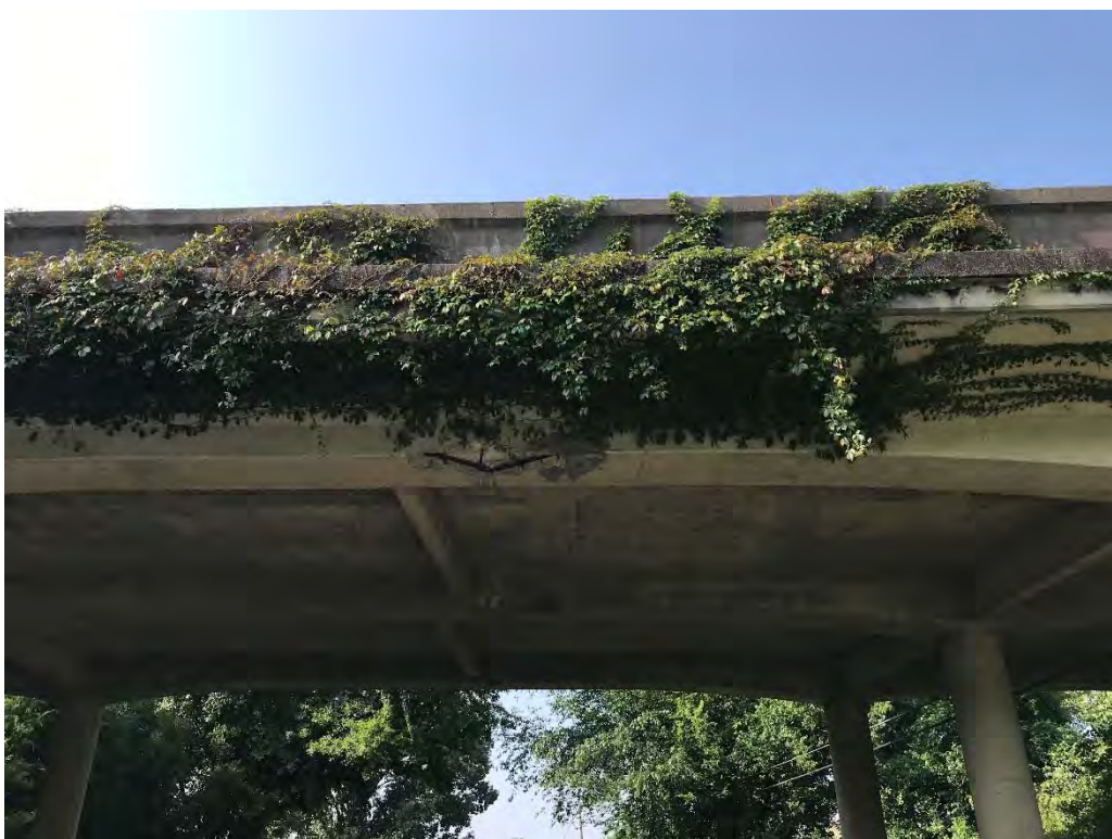
Northern Edge of Bridge
