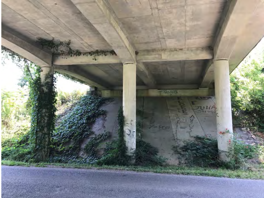
Underside of bridge looking east
