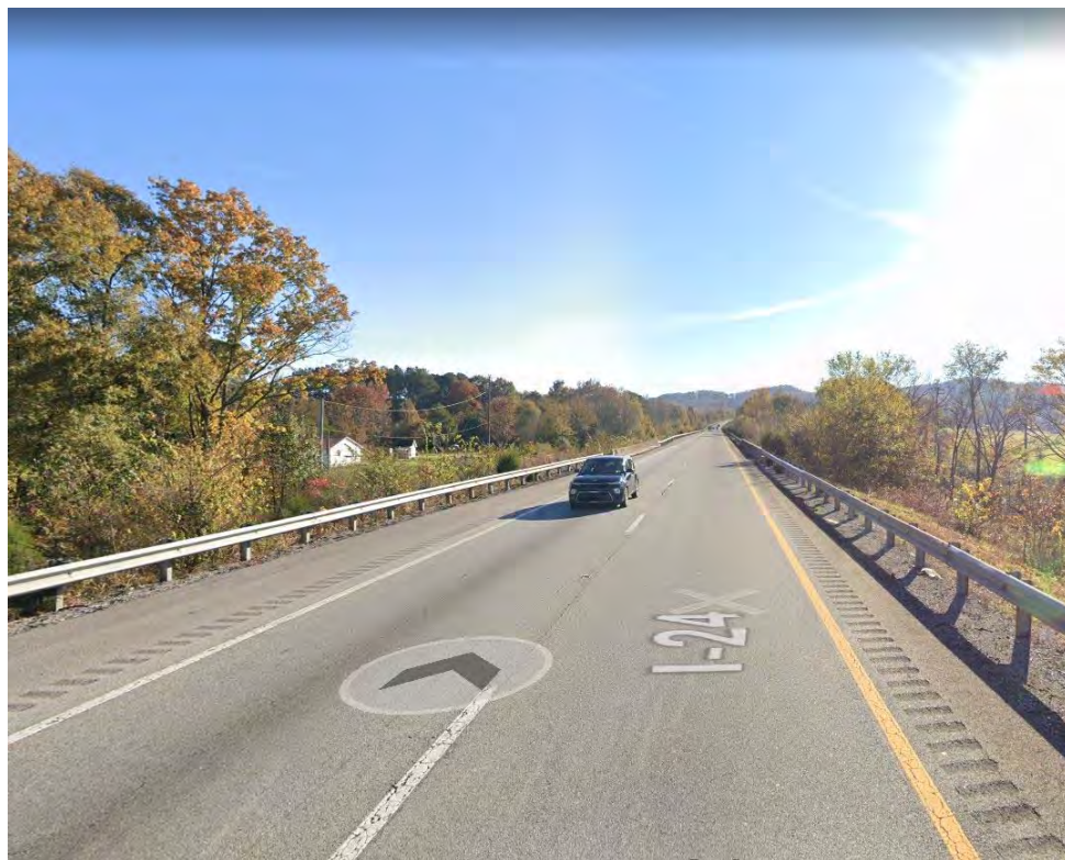
Western Approach Looking East
