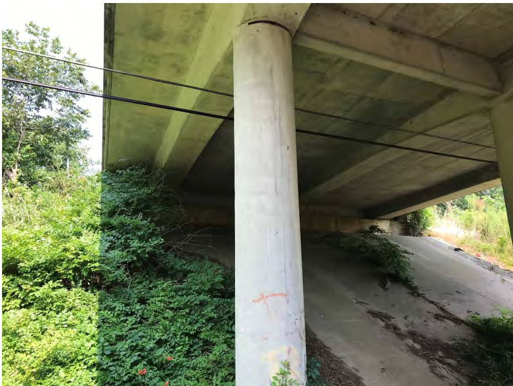
Underside of bridge looking west (featuring utilities)
